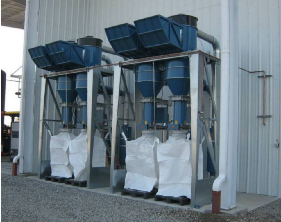
Figure 2.2: Flexfilters 18 EX from Nederman at an industrial workplace.
